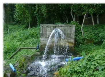
36 cu.m Sump Tank 1 15 LPS Capacity Connected with a 4" Ø Transmission Line
