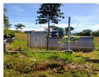
50 cu.m Capacity 625 m above sea level 6" Ø Control Gate Valve (Manila Group) JICA Reservoir With Chlorinator House
