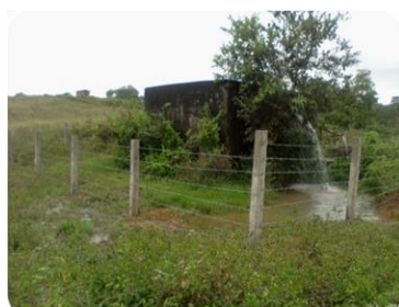
Angelina Reservoir 30 cu.m Capacity 646 m above sea level (Manila Group)
